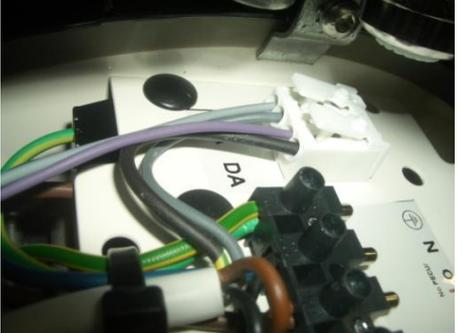
**6.** The RD12 fitting is designed to be used as a post top fitting for 76mm diameter columns. To install, first feed the pre-wired cable into the column and then slowly lower the fitting in place. There are 3 M8 grub screws in the fitting bracket. Once the fitting is in place, start by fully tightening the grub screw closest to the lamp. Once this is fully tightened alternate between the remaining two grub screws, ensuring that the fitting does not lean to one side.
