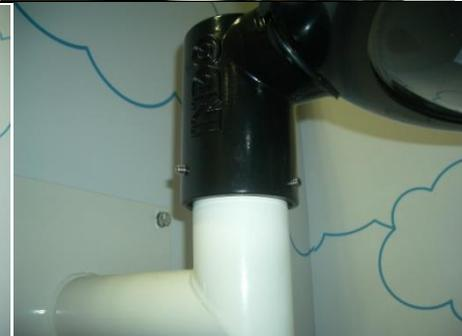
Tighten grub screws to 8-10Nm.
