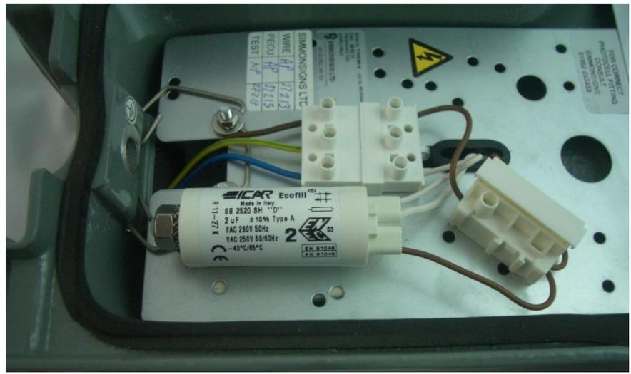
Identify the live-in feed to the capacitor and remove the wire in the fuse block by inserting a small flat blade screwdriver, pull on the wire to release.
