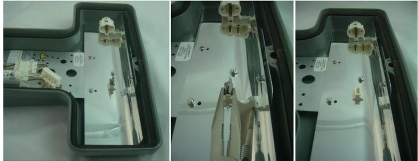
Push the new retaining spring provided into the plastic holder.
