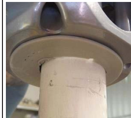
Figure 10 - column sitting against casting
