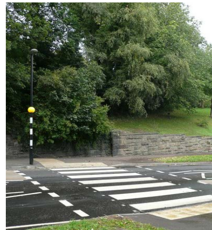
Zebra crossing on two way road with kerbside single Belisha Beacons
